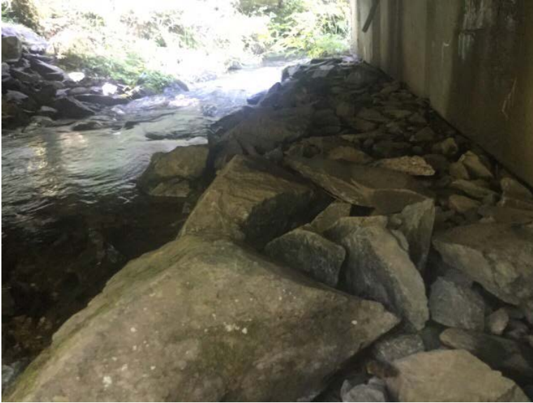
Left Bank Abutment when facing downstream
