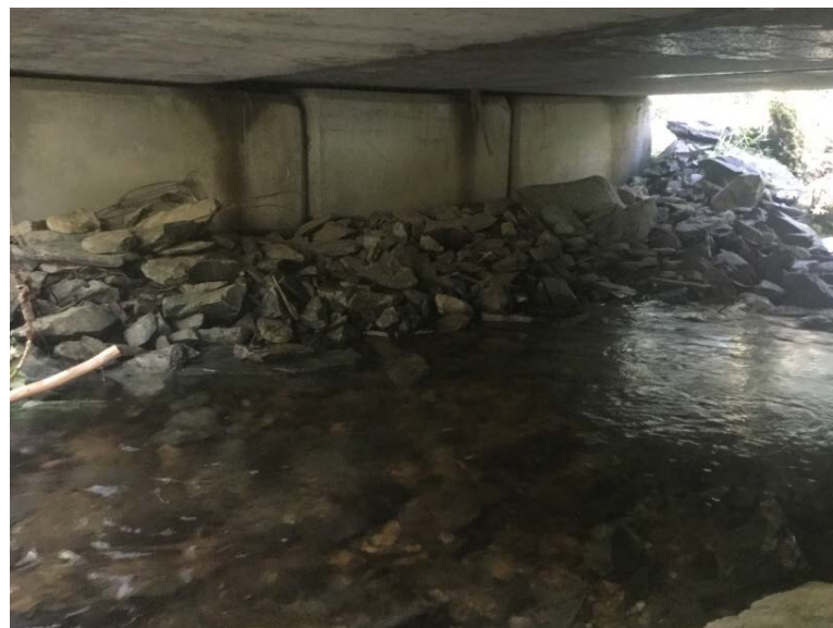
Left Bank Abutment when facing downstream
